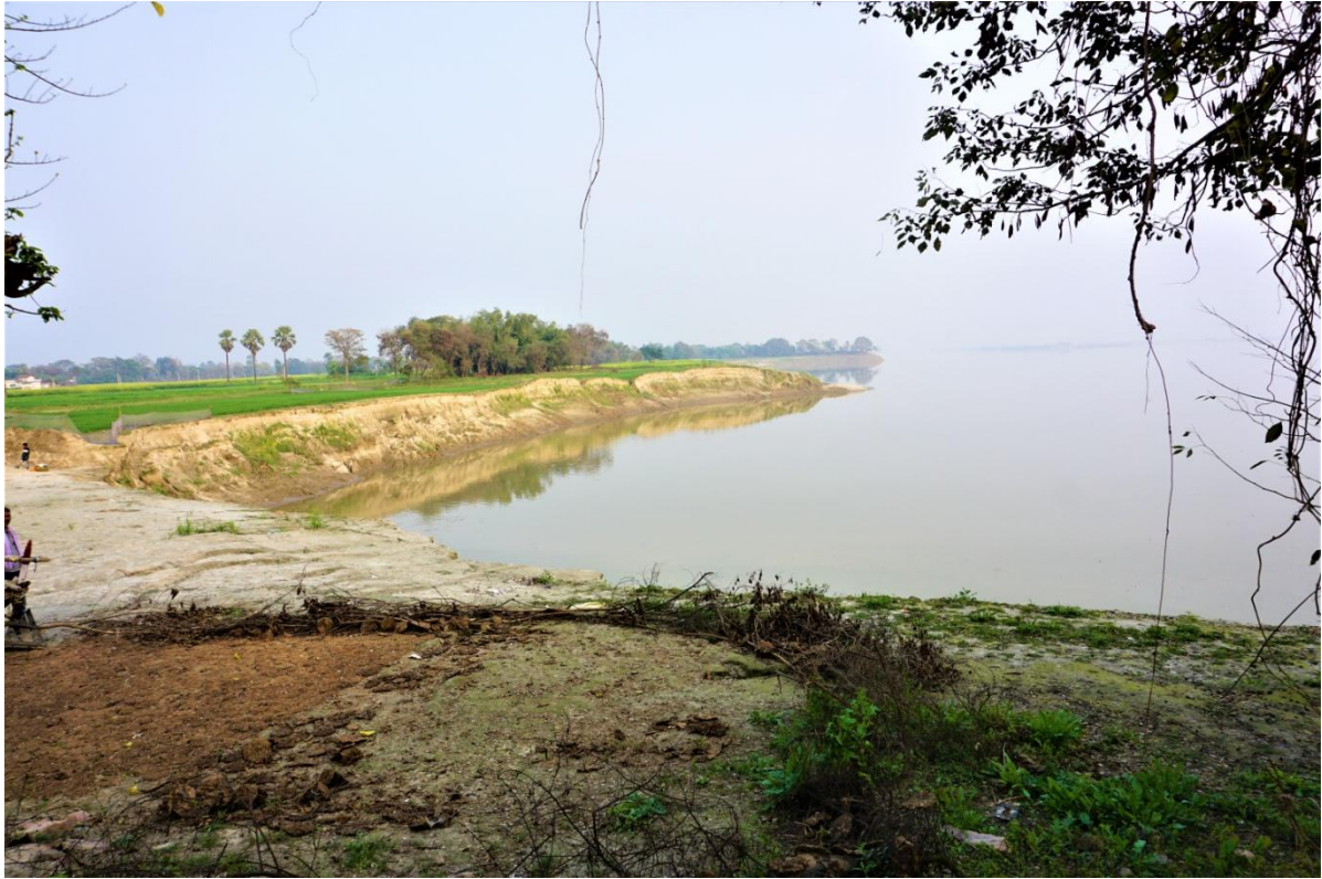
Image 47 : Eroded Bank [Left Bank]
